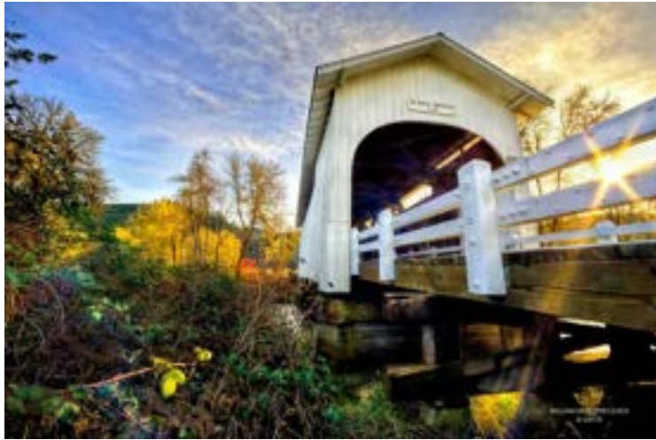
Harris Covered Bridge
