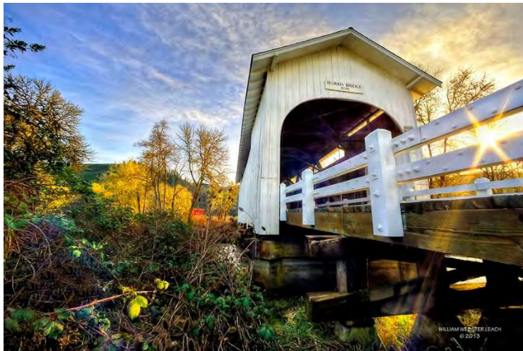
Harris Covered Bridge
