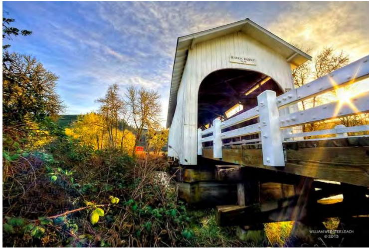
Harris Covered Bridge
